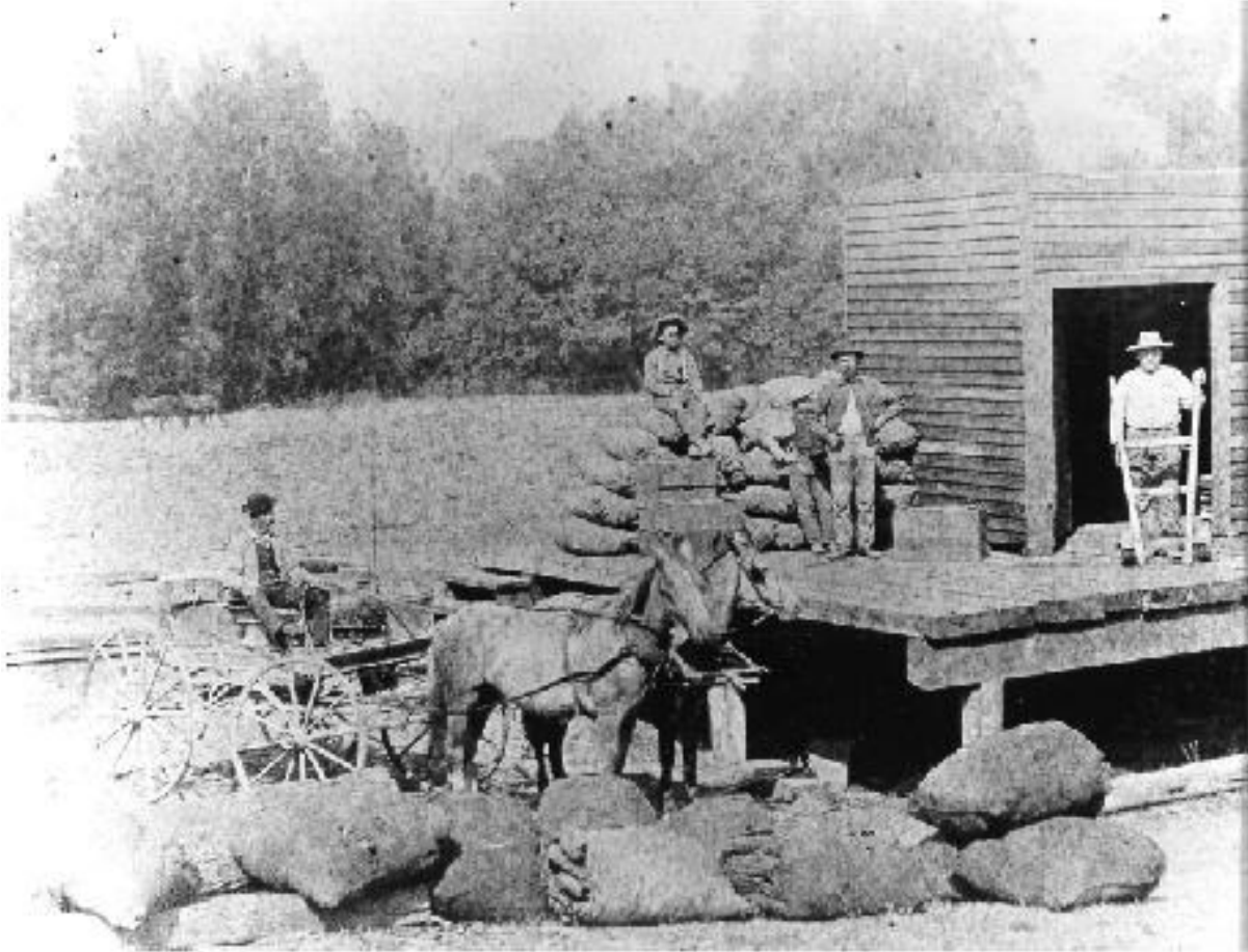
Hauling charcoal to the Northwestern Pacific Railroad Station, Forestville, CA, 1895 (Sonoma County History and Genealogy Library, Photo 7712)
